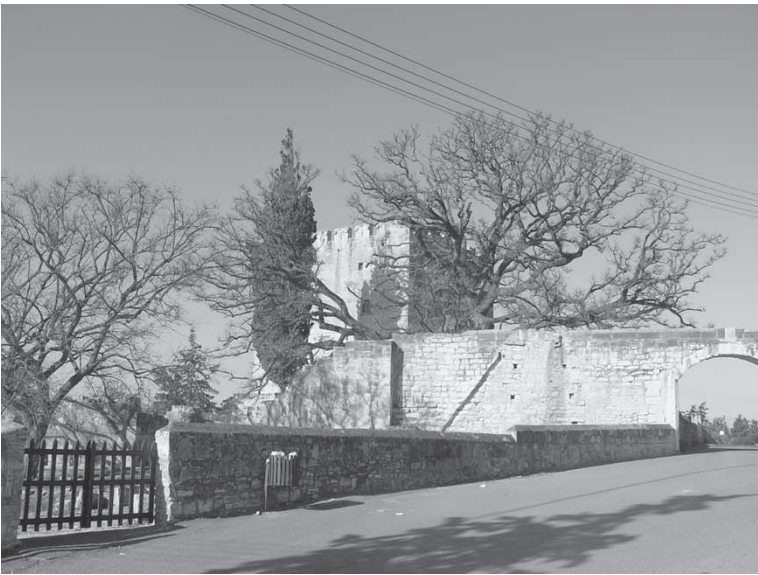
Fig. 72: Kolossi, part of the fourteenth-century aqueduct [M. Olympios].
